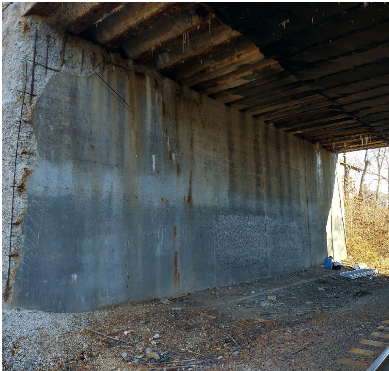
Typical deterioration of bridge abutment
