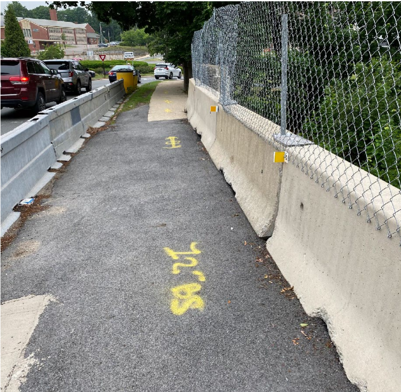
Temporary traffic barriers in place
