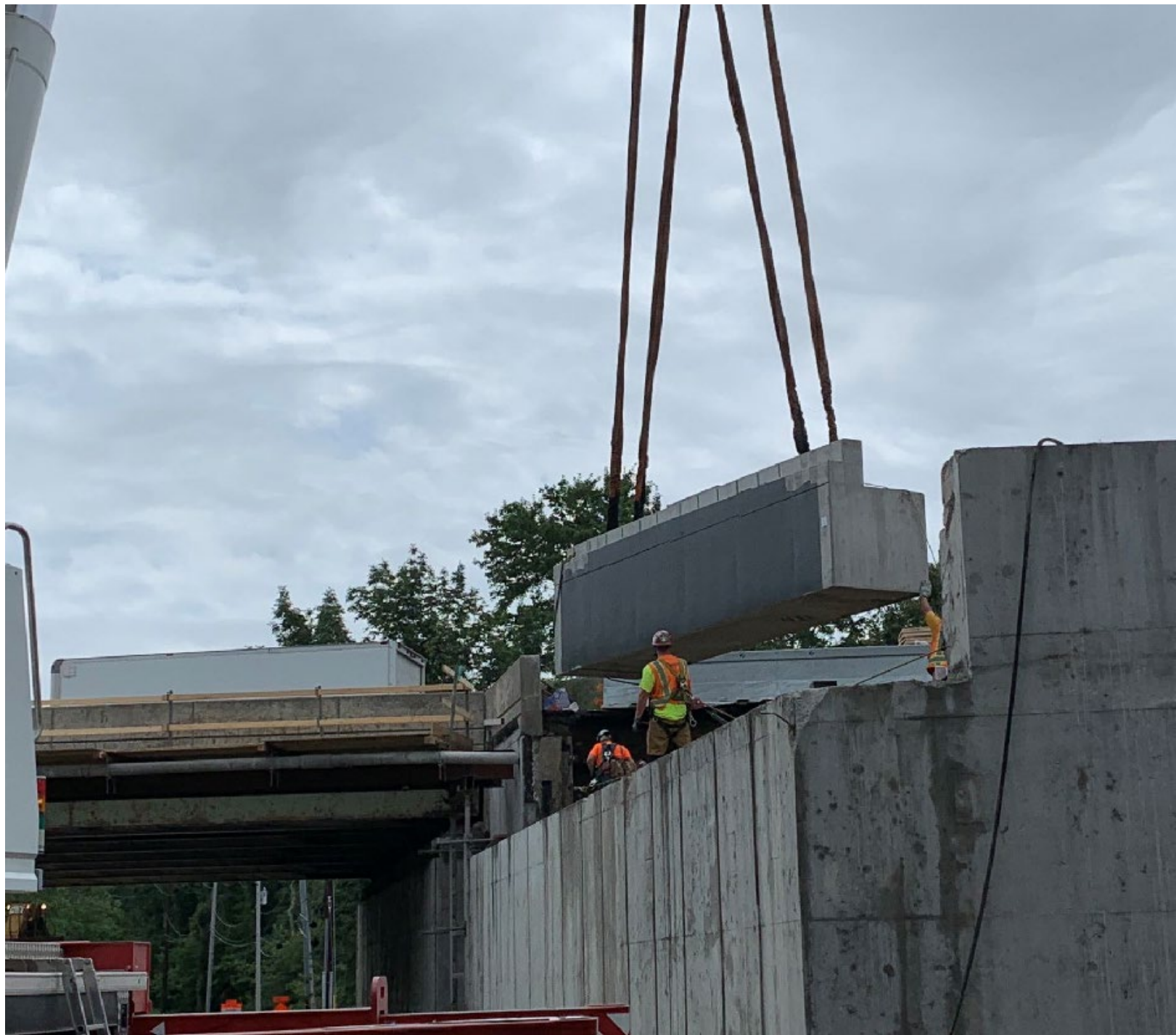
Construction of Precast Abutment Bridge Seat
